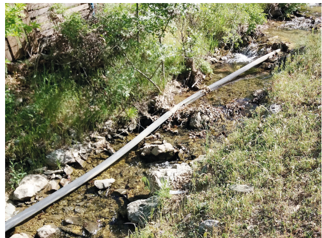
Figure 4. A water pipe draining the stream source for agricultural irrigation.
